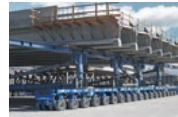
BRIDGE & TUNNEL CONSTRUCTION
